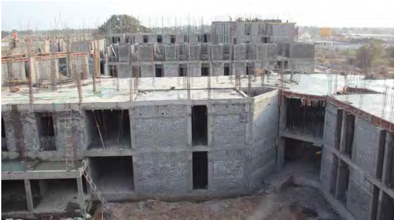
Hostel buildings under construction
