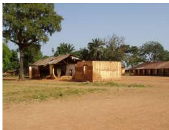
Example of Irrepairable Classroom Building (3)
