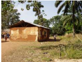
Example of Repairable Classroom Building (2)
