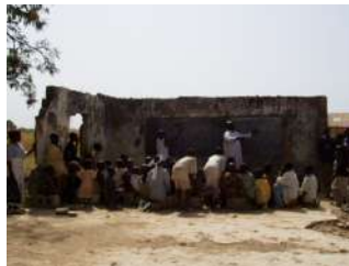
Example of Irrepairable Classroom Building (1)
