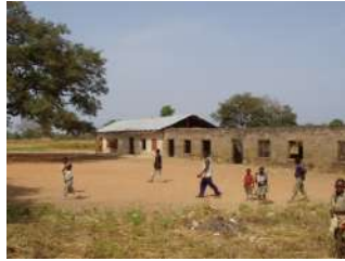
Example of Repairable Classroom Building (1)
