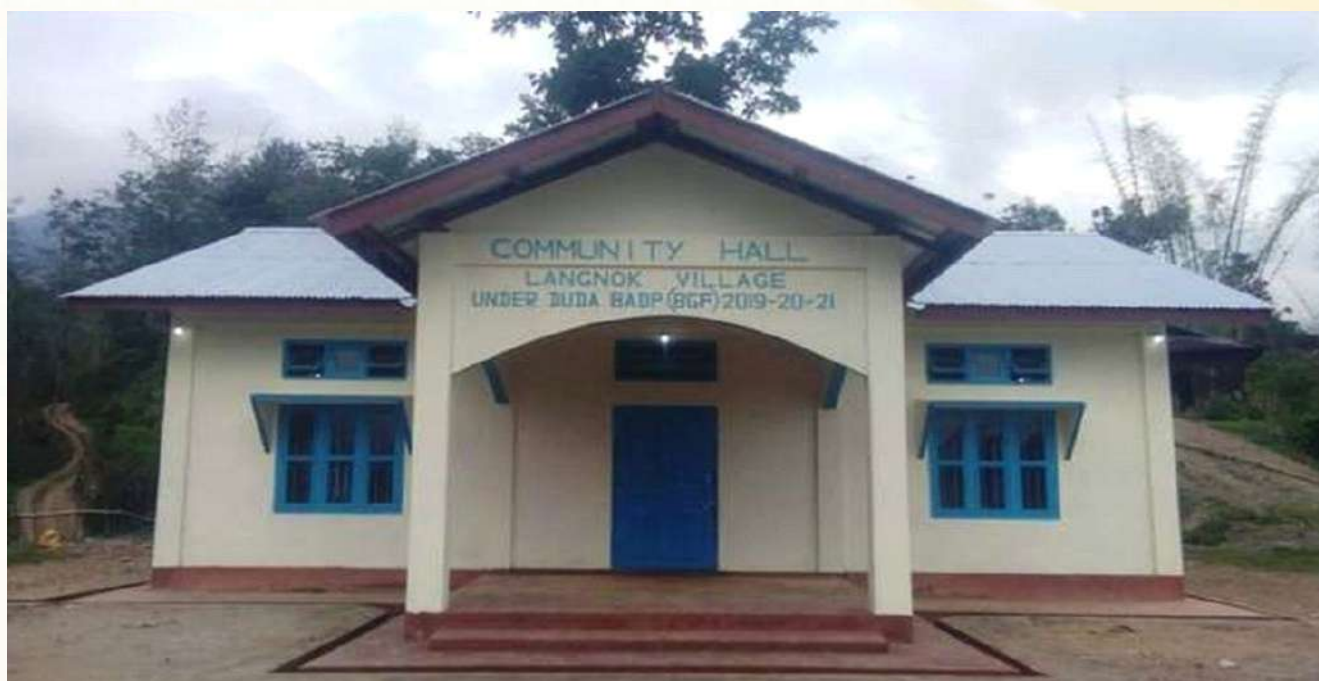
Construction of community hall at village- Langnok, District-Noklak, Nagaland. Date of completion of the work: 12.08.2021
