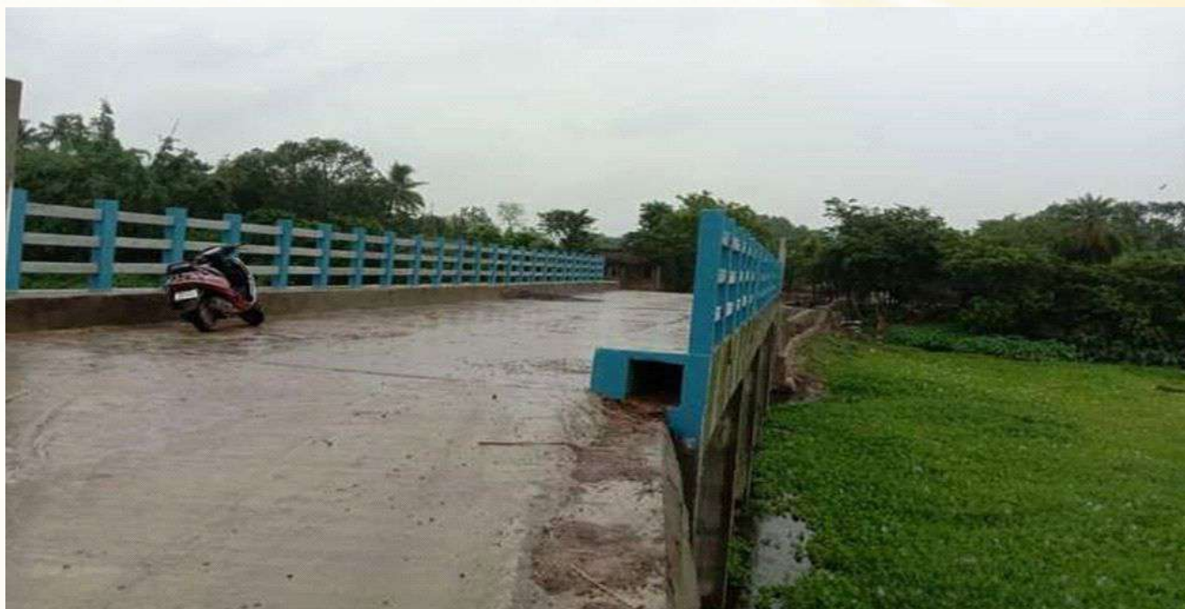
Construction of Major Culvert on river Bhairab with approach road at Village - Habaspur Moti Mahal under Block - Bhagwangola-I, Distt - Murshidabad, West Bengal. Date of completion of the work - 15.06.2021.
