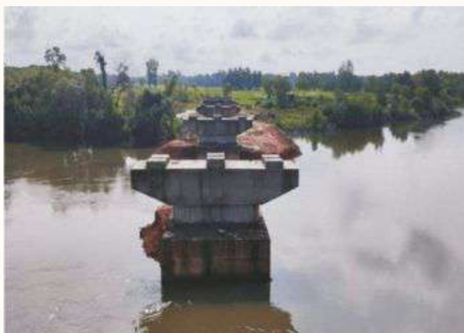
Bridge work under progress at Udupi, Karnataka
