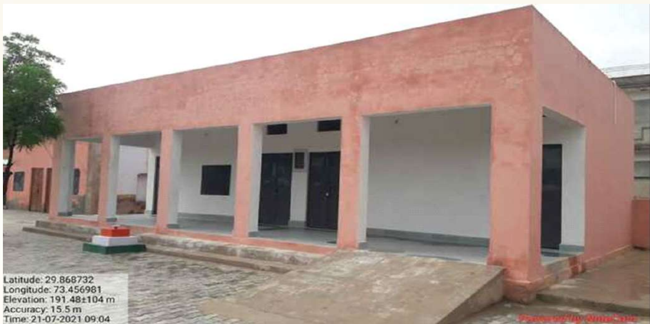
Construction of two rooms with Verandah in Govt. Primary School at Village -17 O, Block- Sri Karanpur, District – Sri Ganganagar, Rajasthan. Date of completion: 15.05.2021
