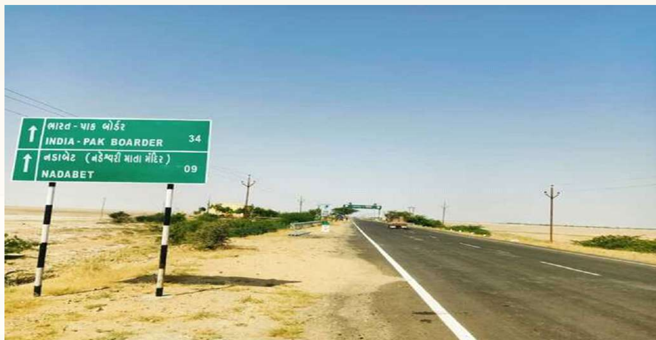
Construction, Widening & Strengthening of Suigam Jaloya Nadabet Road (km 0/000 to 19/600), Teh. Suigam, Distt. Banaskantha, Gujarat. Date of completion 26.02.2021
