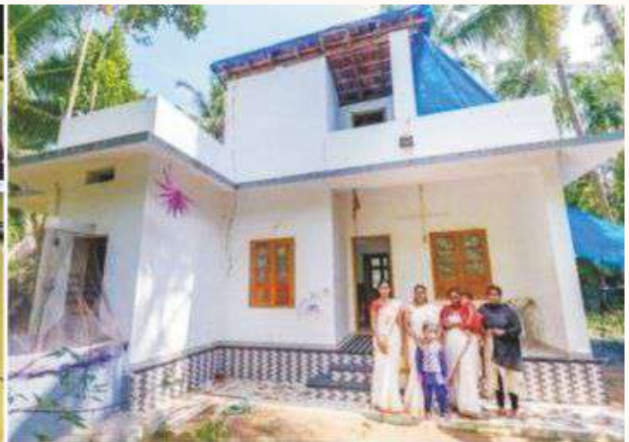
Construction of houses under PMAY
