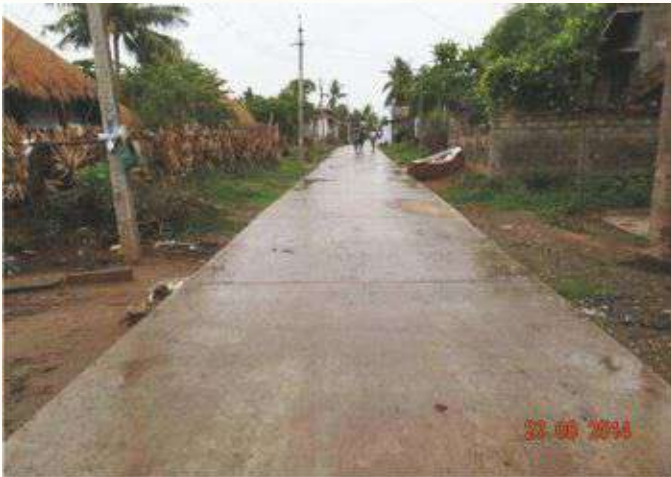
Road at Dindi, Andhra Pradesh
