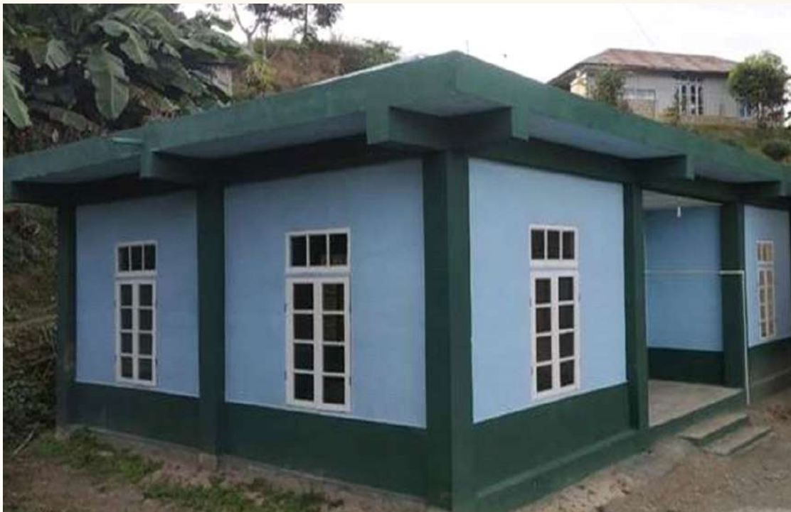
Construction of Health Sub-Centre building at Village-South Vanlaiphai, Block-Hnahthial, District -Hnahthial, Mizoram. Date of completion of the work - 22.03.2021.
