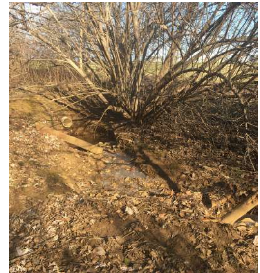
Pipe outfall at center of wetland area
