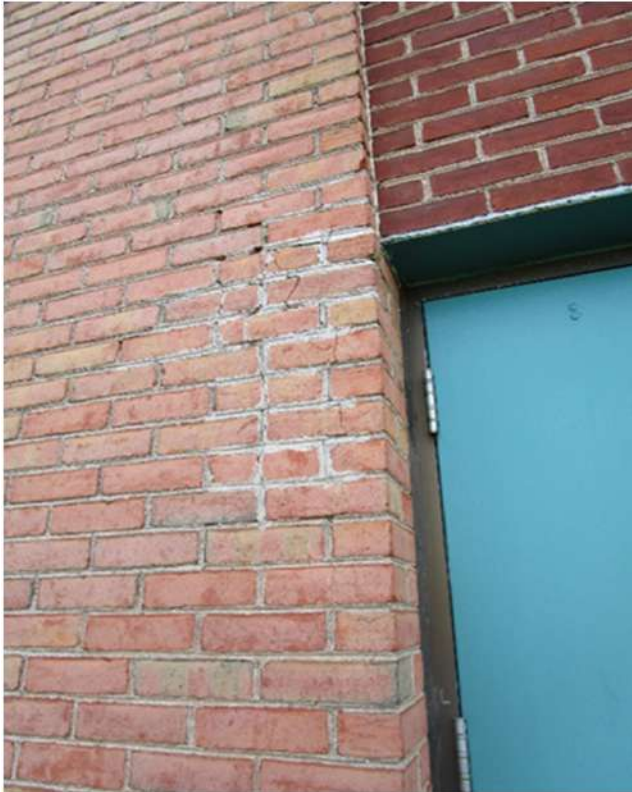
Photos 4A and 4B: Second Classroom Wing East side lintels – replace lintel beam and masonry jambs
