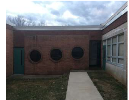
Connection between central wing and classroom addition
