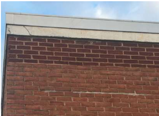
Mortar joint repairs, cracking marble course
