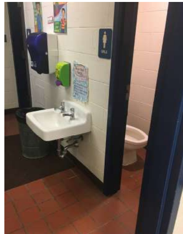
Single-user toilet rooms are not ADA compliant due to size and door width
