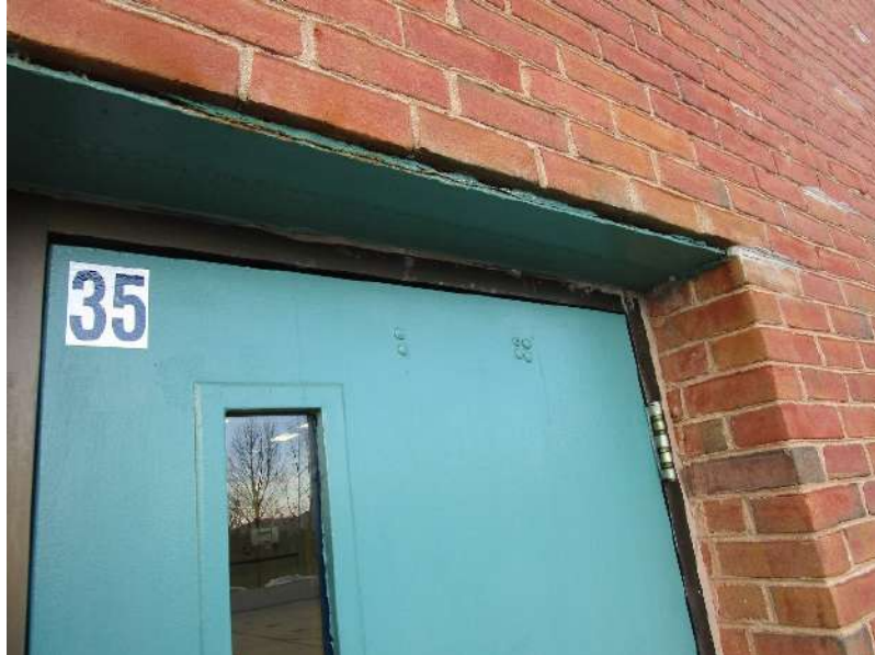
Photos 5A and 5B: Gym and gym vestibule lintels – replace lintel beam and angles
