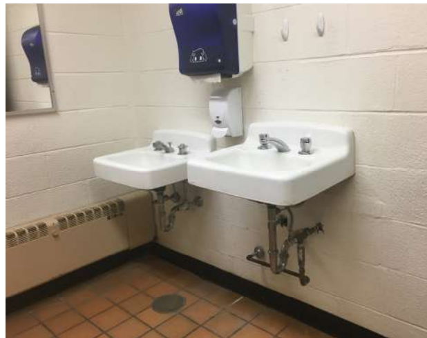
Multi-user restroom with painted CMU walls, ceramic tile flooring, and vinyl base
