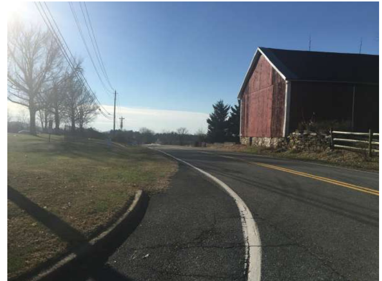
View to south along Horine Road with slight crown
