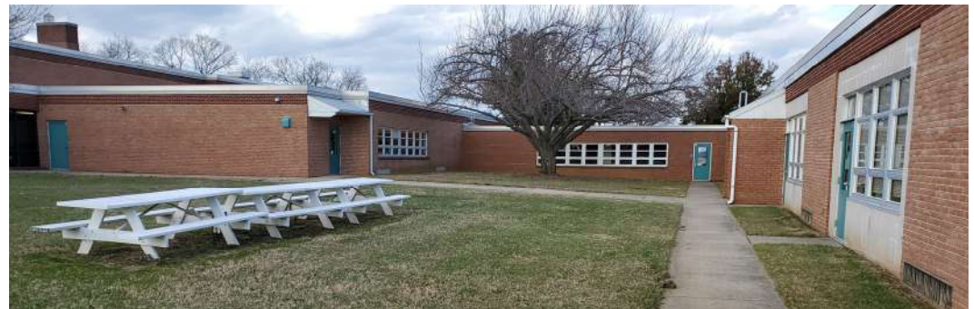
South side of art room and connector link between assembly area and classrooms
