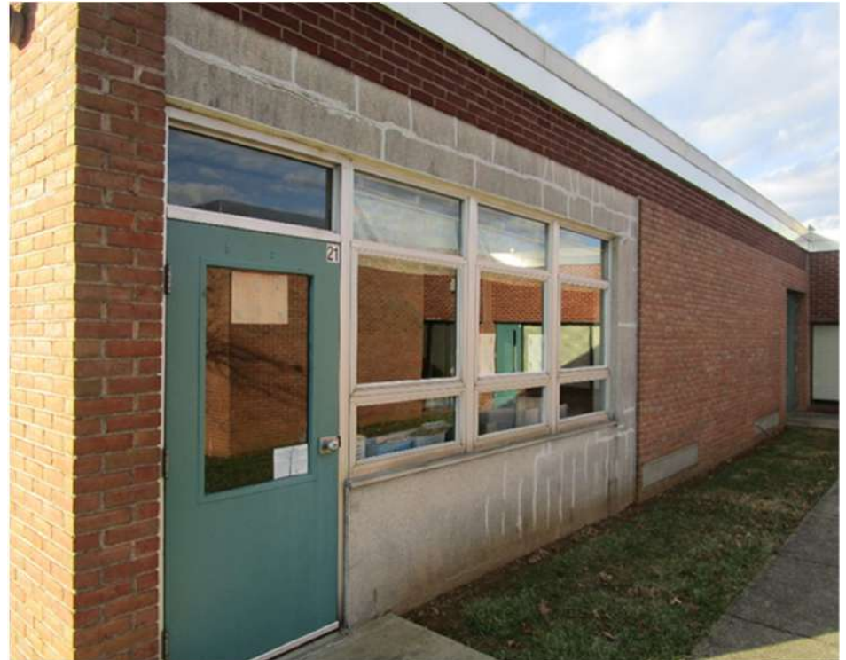
Photo 3: First Classroom Wing East corner lintels – replace lintel beam
