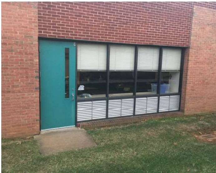
1973 addition typical exterior door & windows
