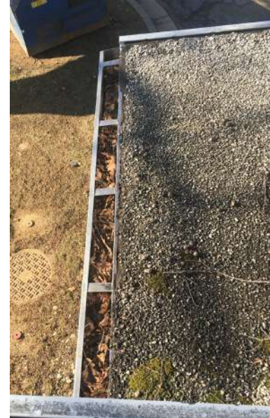
Loading Dock gutter
