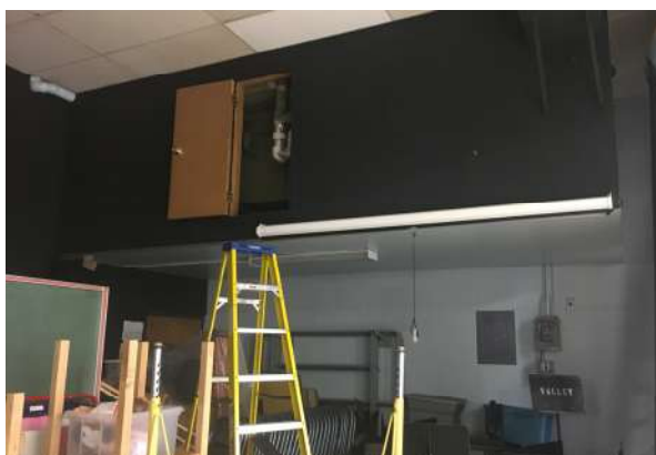
Access door to mechanical platform above stage
