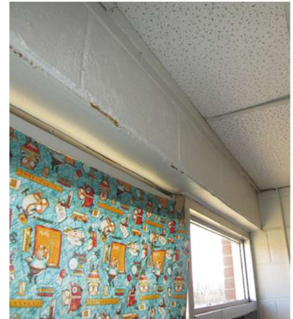
Photos 1A and 1B: First classroom Wing – Steel Lintel and CMU jamb damage
