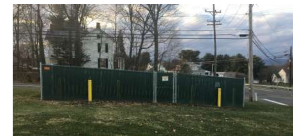
Washington Gas pipeline gateway
