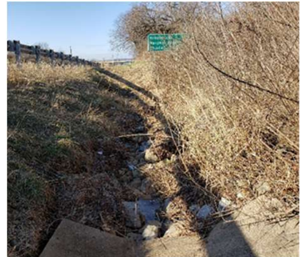
US-340 westbound drainage channel
