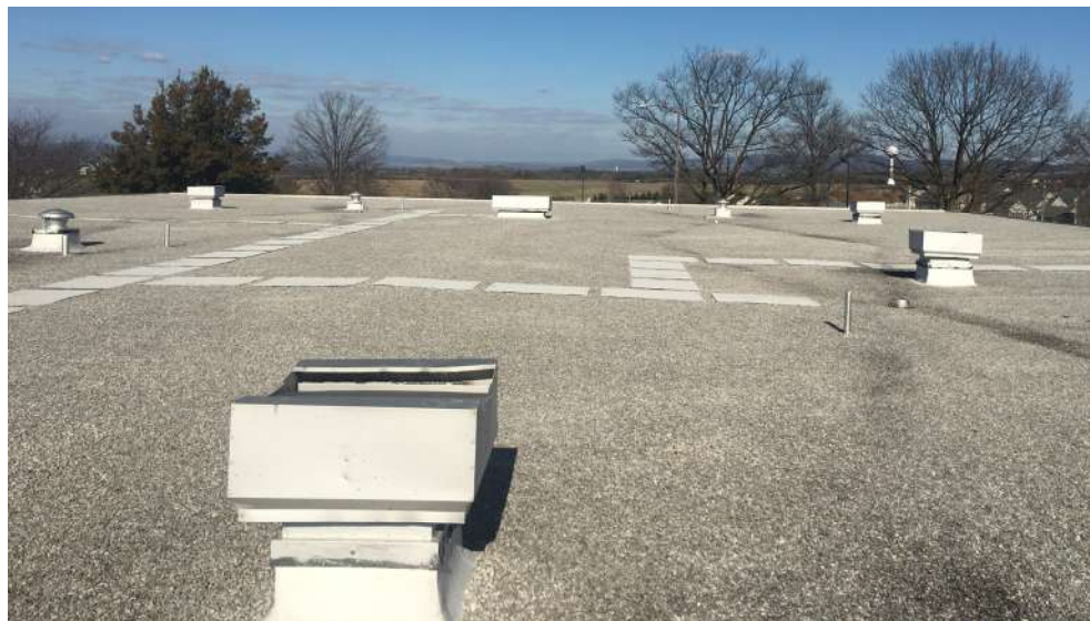
Overview of built-up asphalt roof at original construction classroom wing
