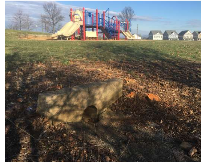
Pipe outfall at top of wetland area
