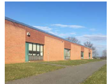
1973 Classroom addition east elevation
