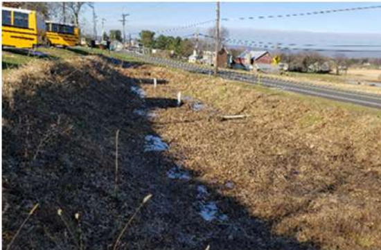
View of SWM facility along Jefferson Pike
