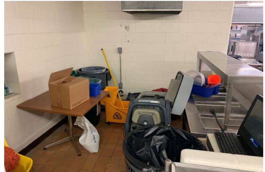
View of dishwashing area with equipment removed
