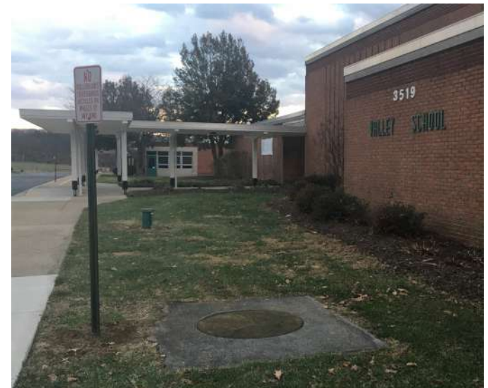
Existing well and underground tank to north of school
