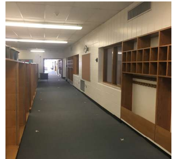
View of makeshift west media corridor
