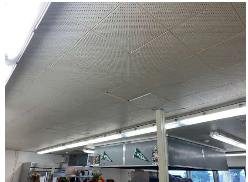
View of perforated ceiling tile
