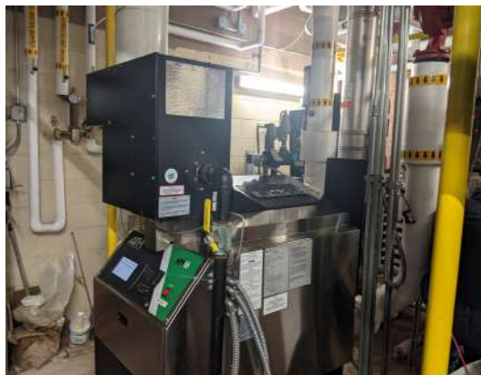
High-efficiency condensing-type boiler
