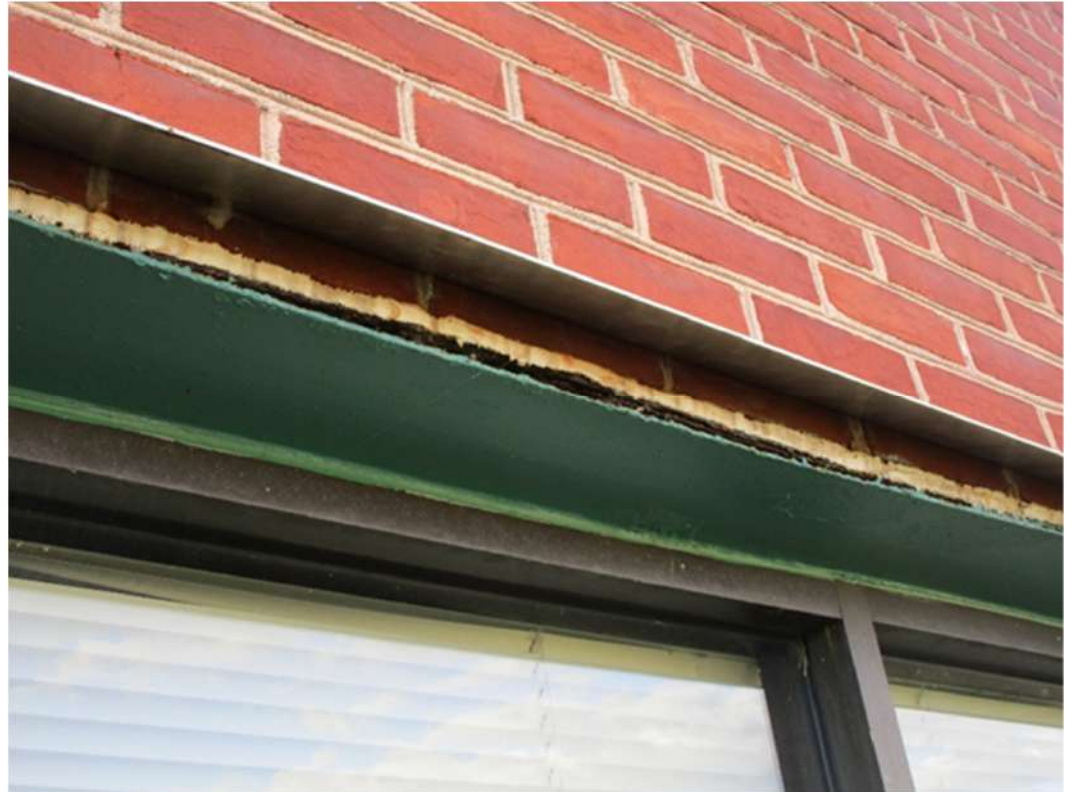
Photos 4A and 4B: Second Classroom Wing East side lintels – replace lintel beam and masonry jambs
