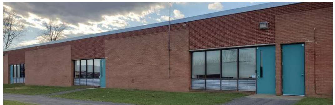
East side of classroom addition
