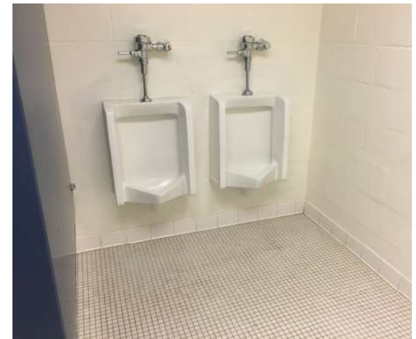
Multi-user restroom with painted CMU walls, ceramic tile flooring, and tile base
