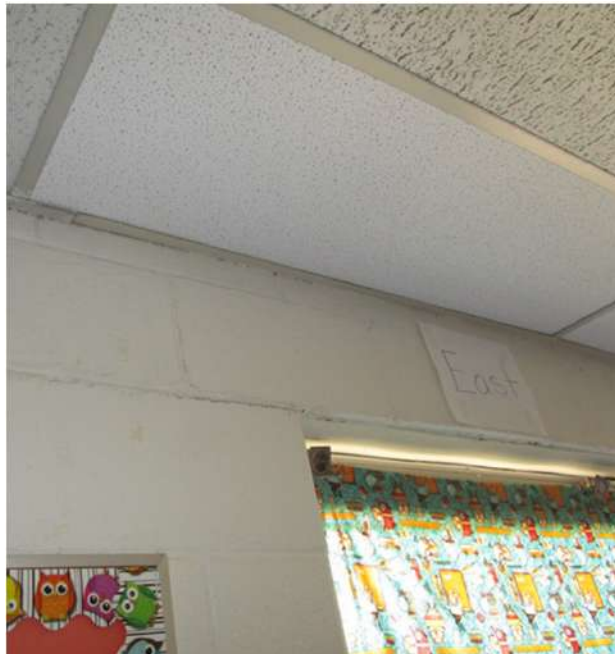
Photos 1A and 1B: First classroom Wing – Steel Lintel and CMU jamb damage
