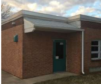
Asphalt shingle overhang
