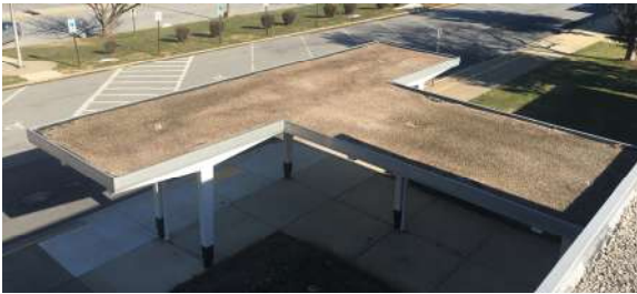
Main entry canopy roof
