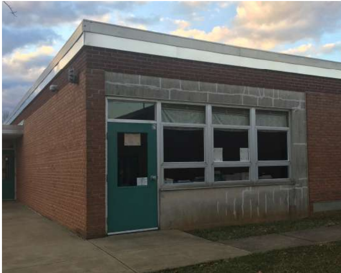
Original building typical classroom exterior door/window
