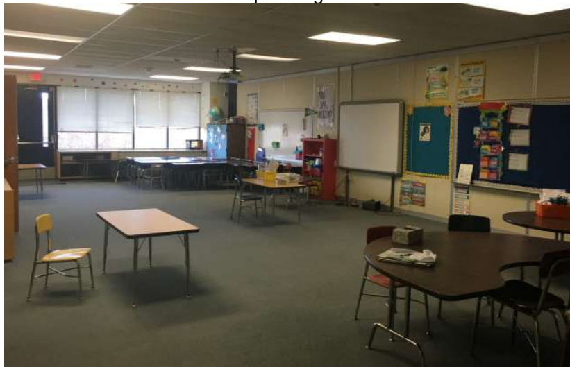
Typical addition wing classroom with demountable wall
