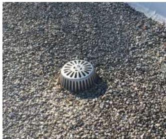
Classroom wing roof drain
