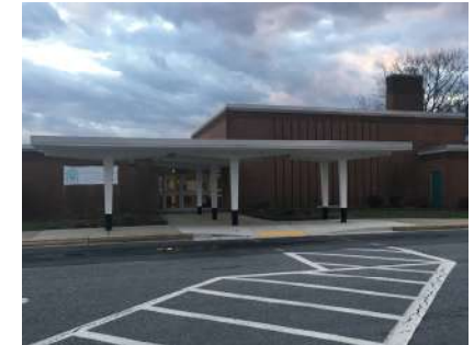
View of main entrance canopy from parking lot
