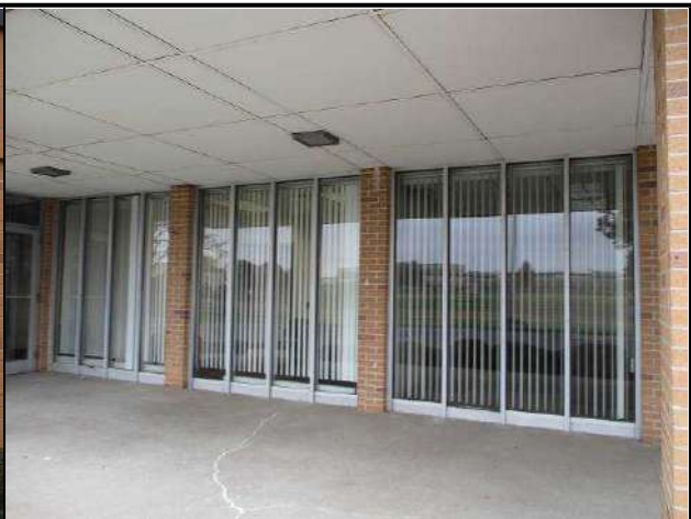
Typical storefront system at tenant entrances.
