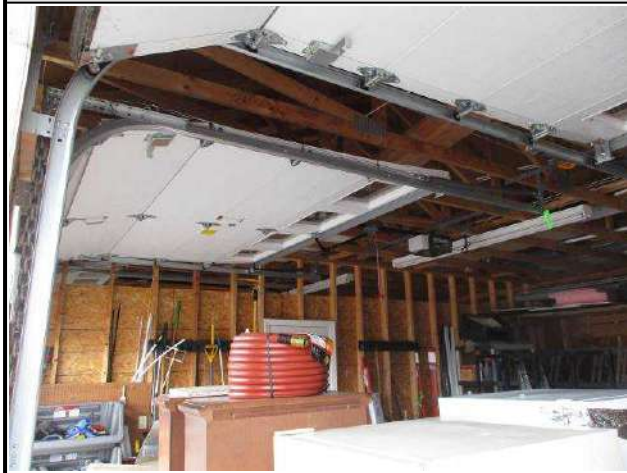
Maintenance garage building overhead doors.
