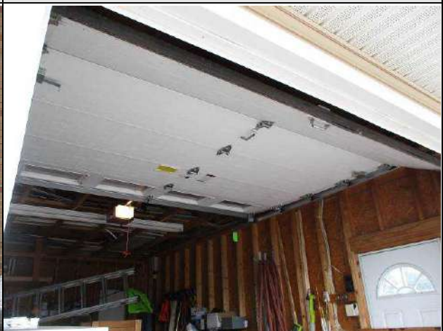
Typical overhead sectional garage door.
