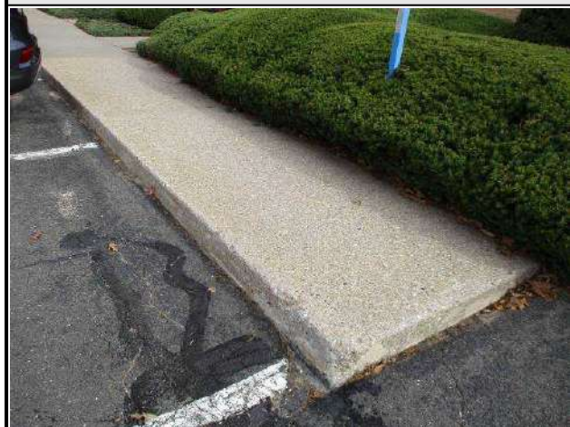
Typical concrete sidewalks.
