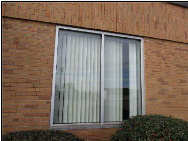
Typical fixed, punched, aluminum-framed window.
