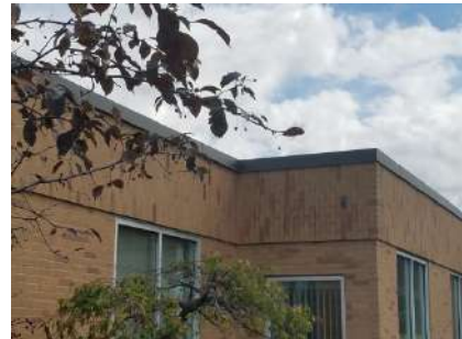
Roof is low sloping with no parapet.
