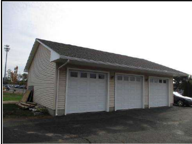
Maintenance garage building front and north side.
