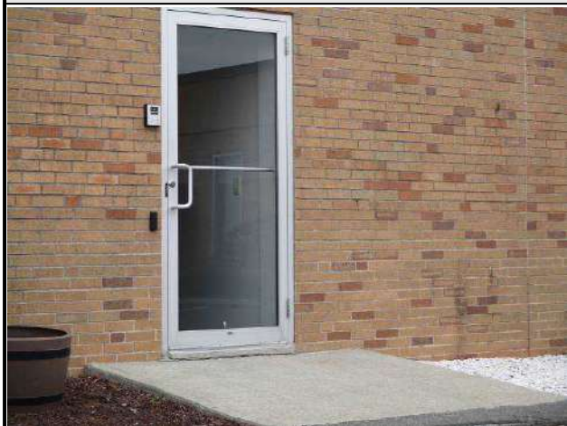
Typical aluminum and glass door.
