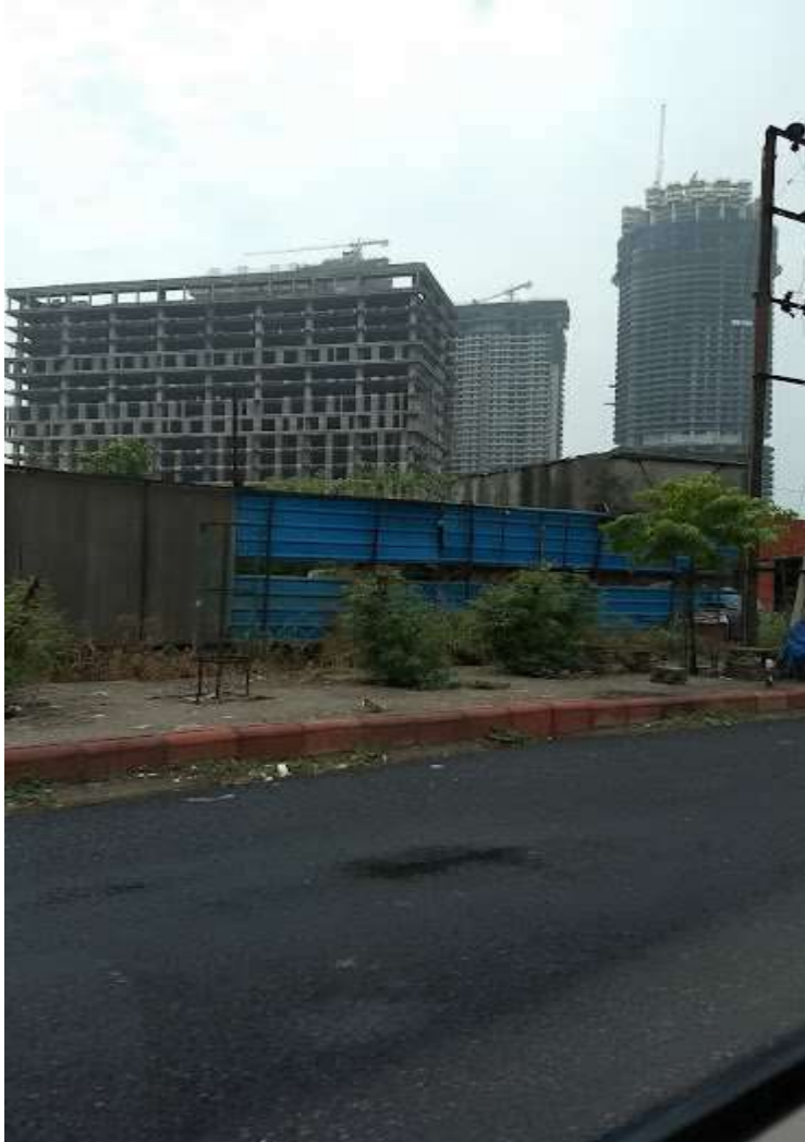
Semi-constructed buildings in Gurgaon, June 2017. By 2018, these offices were being rented by startup companies and coworking spaces. Photograph by author.
