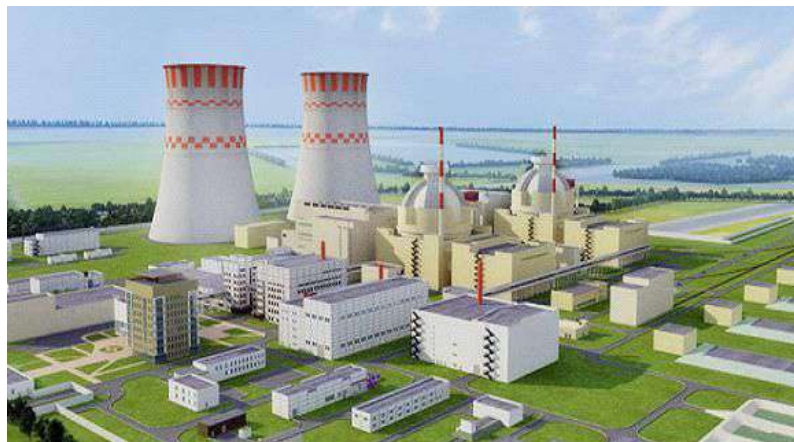
Rooppur Nuclear Power Plant
