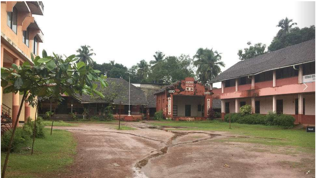
Before- Entry Side
