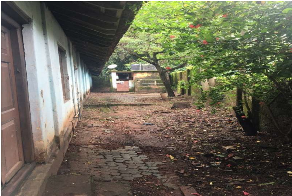
Before- Backside of Building
