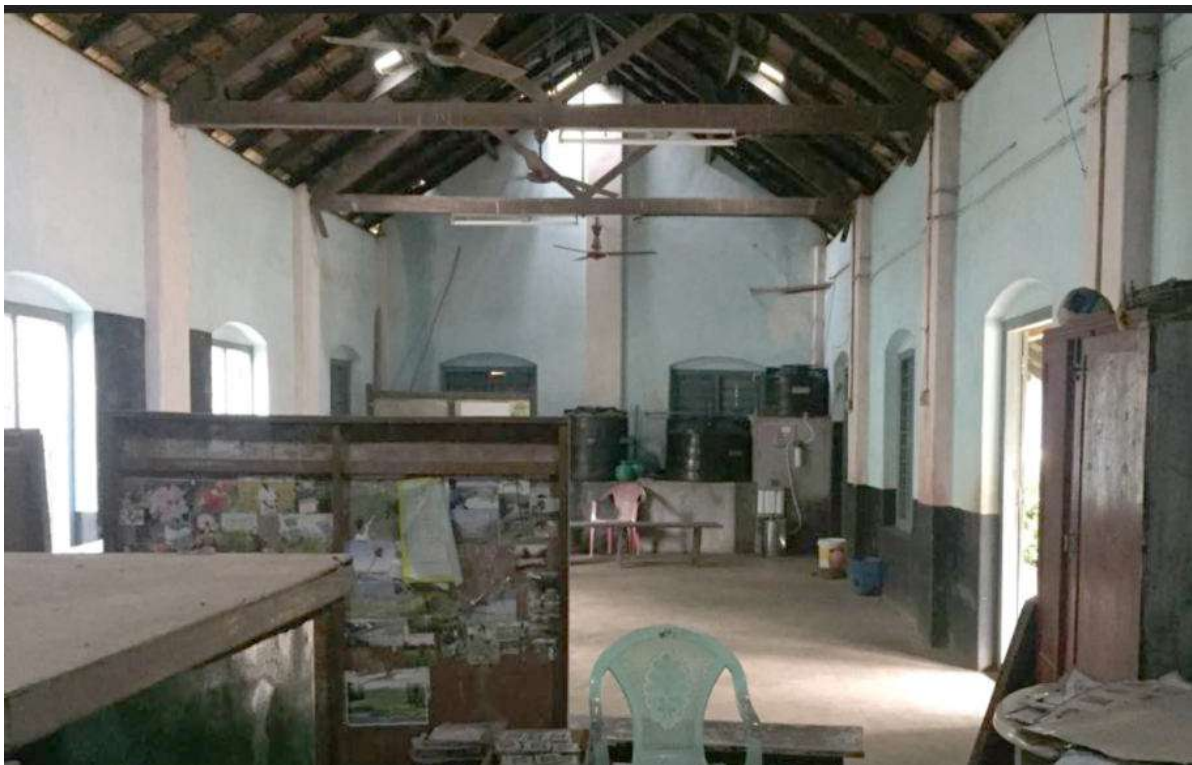
Before- Inside Classroom
