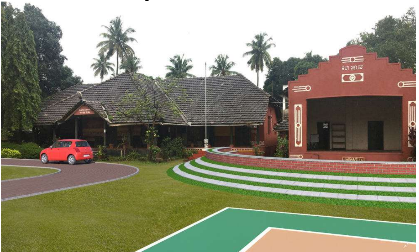
After- Front of Admin Block & Stage
