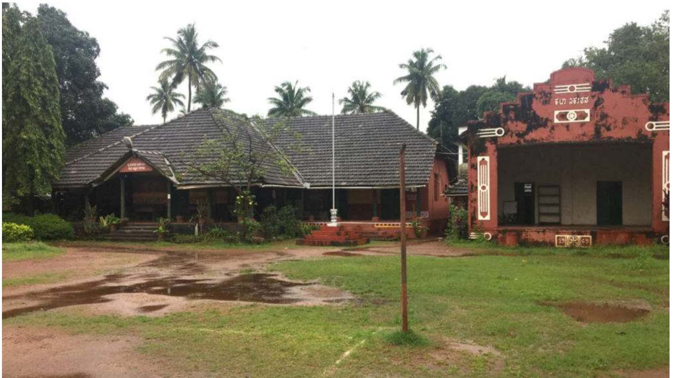
Before- Front Of Admin Block & Stage
