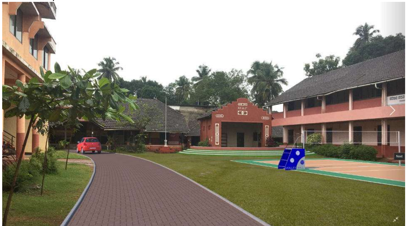
After- Entry Side
