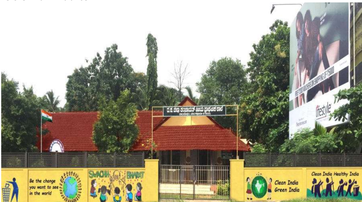
After- Main Entrance
