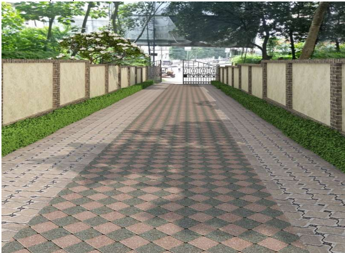
After- Entry Ramp
