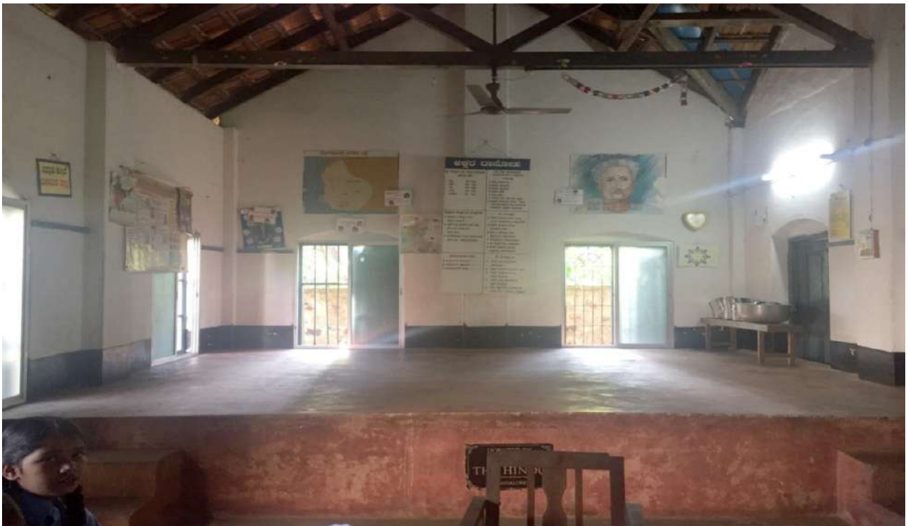
Before- Classroom With Stage
