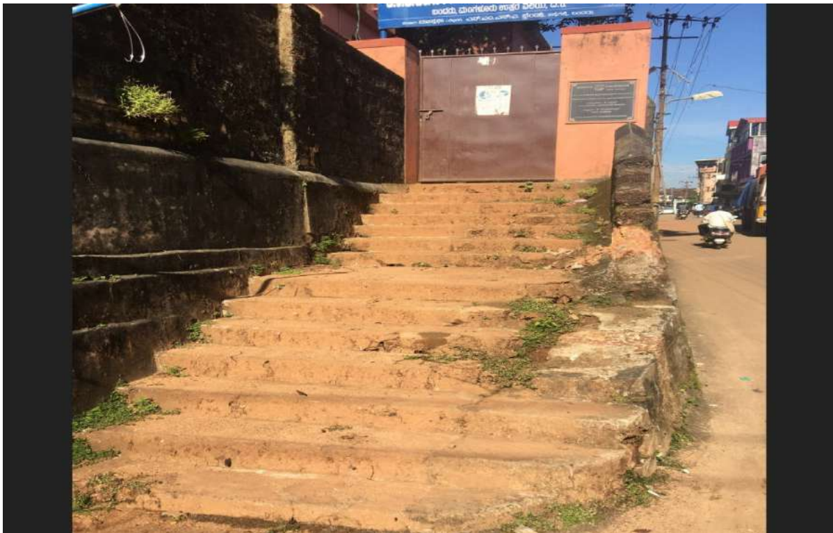
Before- Existing Gate
